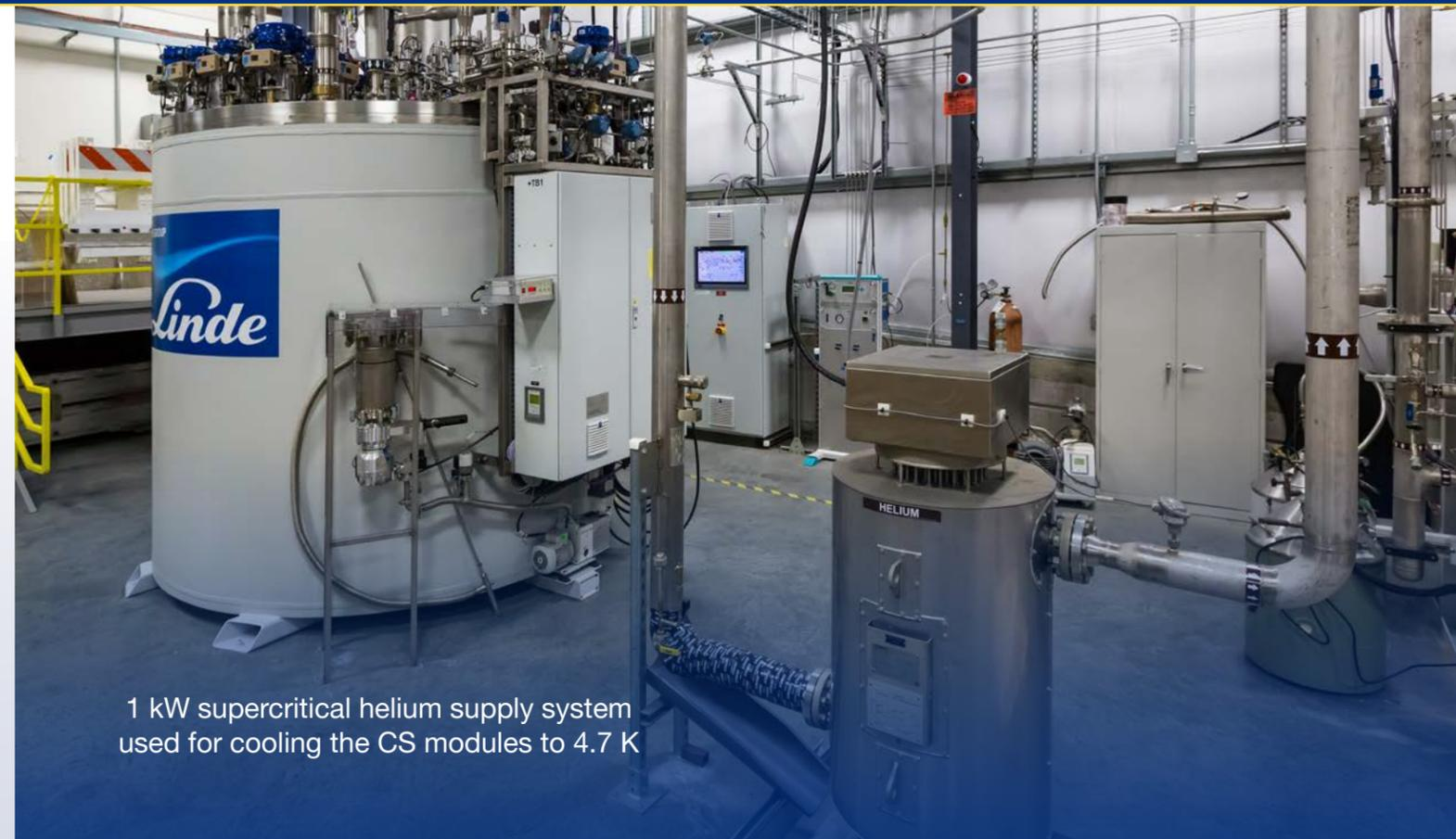
1 kW supercritical helium supply system used for cooling the CS modules to 4.7 K
