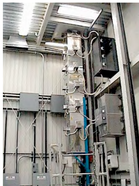
Glass drop tower.
