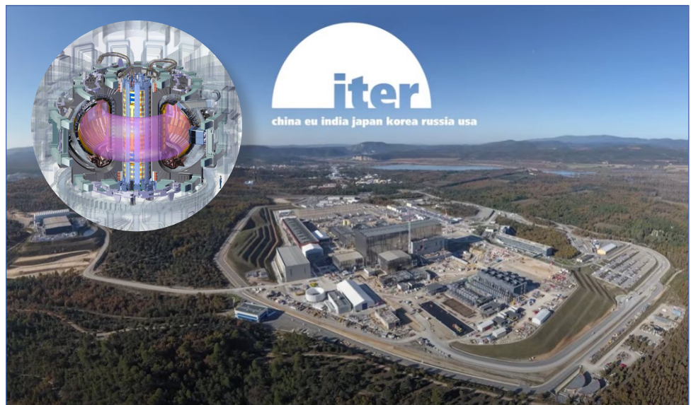
Construction of the ITER project in France is now 75% complete with first plasma scheduled for 2025. Courtesy ITER
