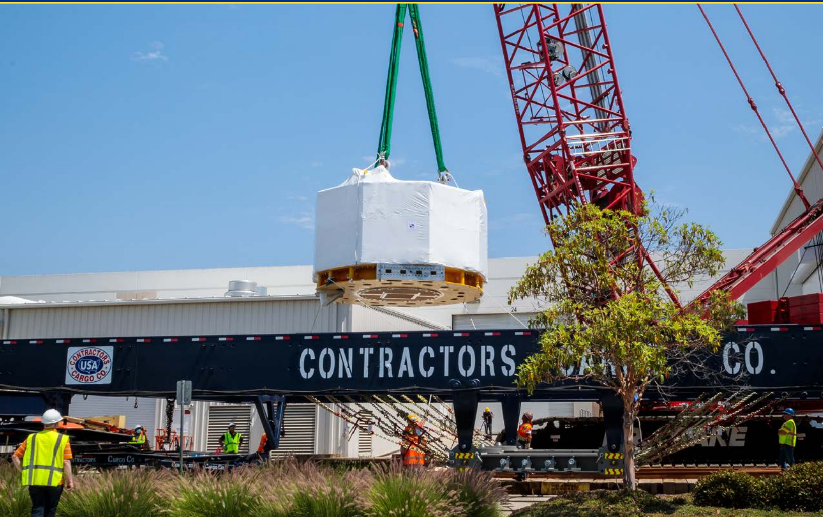
Lowering module into the 24-axle super-heavy trailer
