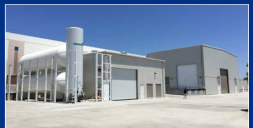
Final Test Facility
