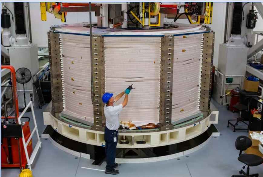
Turn insulation of module nearing completion
