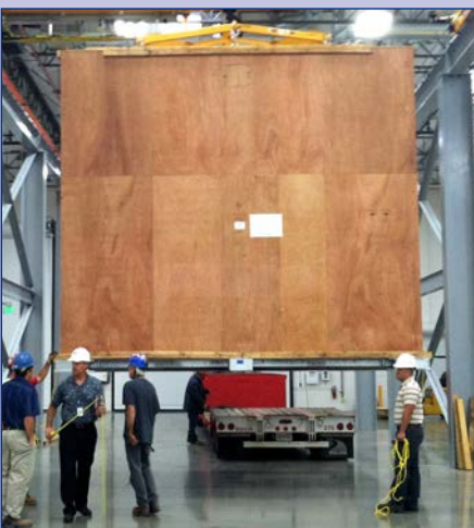
Unloading a conductor spool from the delivery
