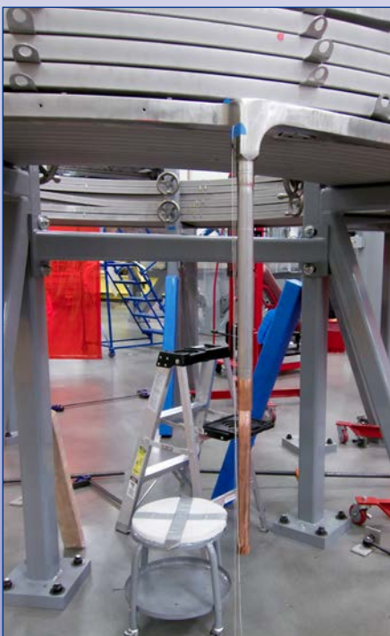
Terminal lead nearing completion
